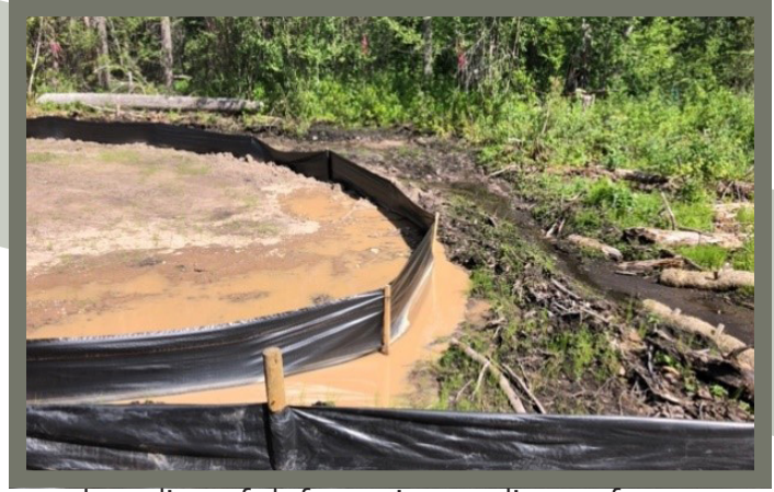
Last line of defense is a sediment fence
