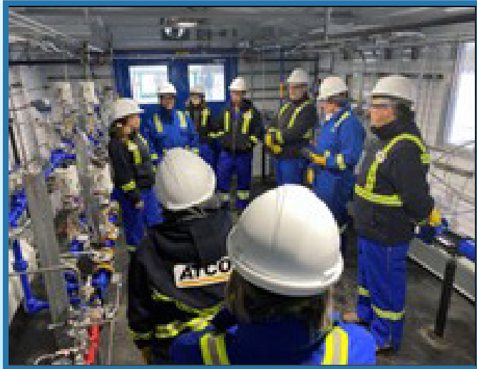
Figure 3. Fort Saskatchewan Hydrogen blending facilities
